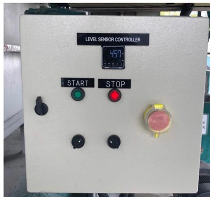
Figure 4: Ultrasonic level sensor controller.
