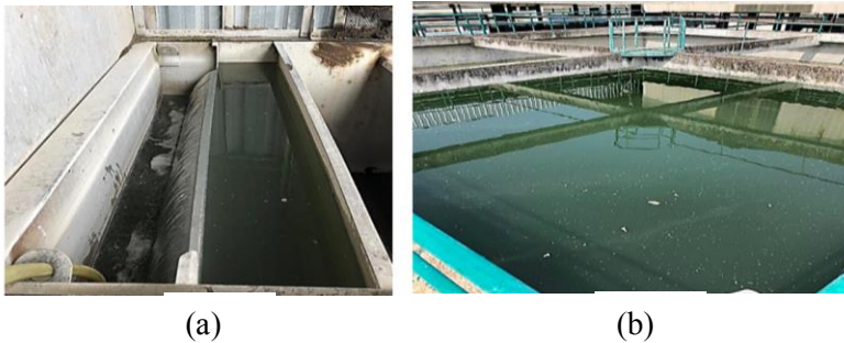
Figure 5: Improvement of retrofitting (a) No suspended carry- over at the Dissolved Air Flotation Chamber. (b) Clear water and good sludge settling at the sequential batch reactor.
