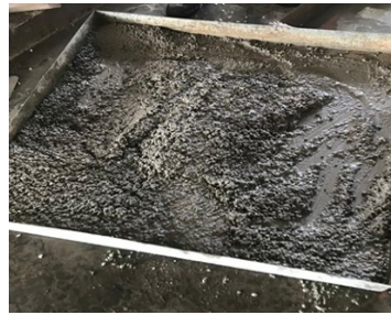
Figure 5: Well mixed concrete mixture
